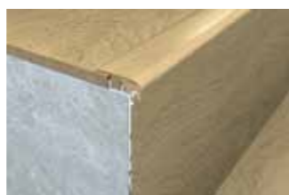
Transition between the top step and the rest of your floor.
